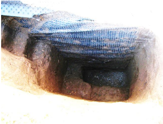
Fig. 12.1 Manually dug trench.
