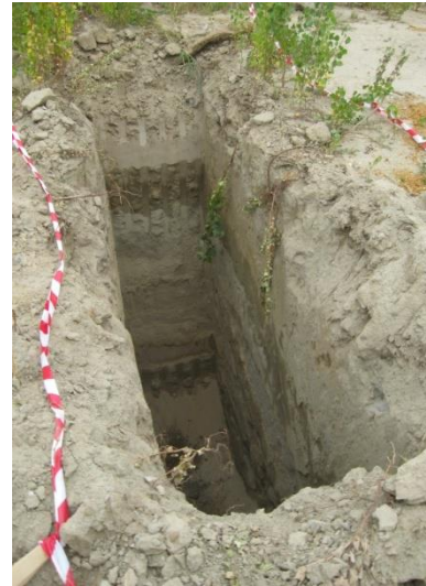
Fig. 12.2 Mechanically excavated trench.
