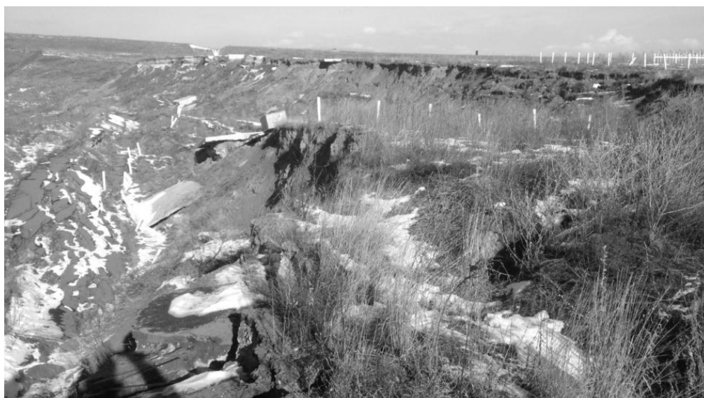
Figure 4. Picture of the actual landslide
